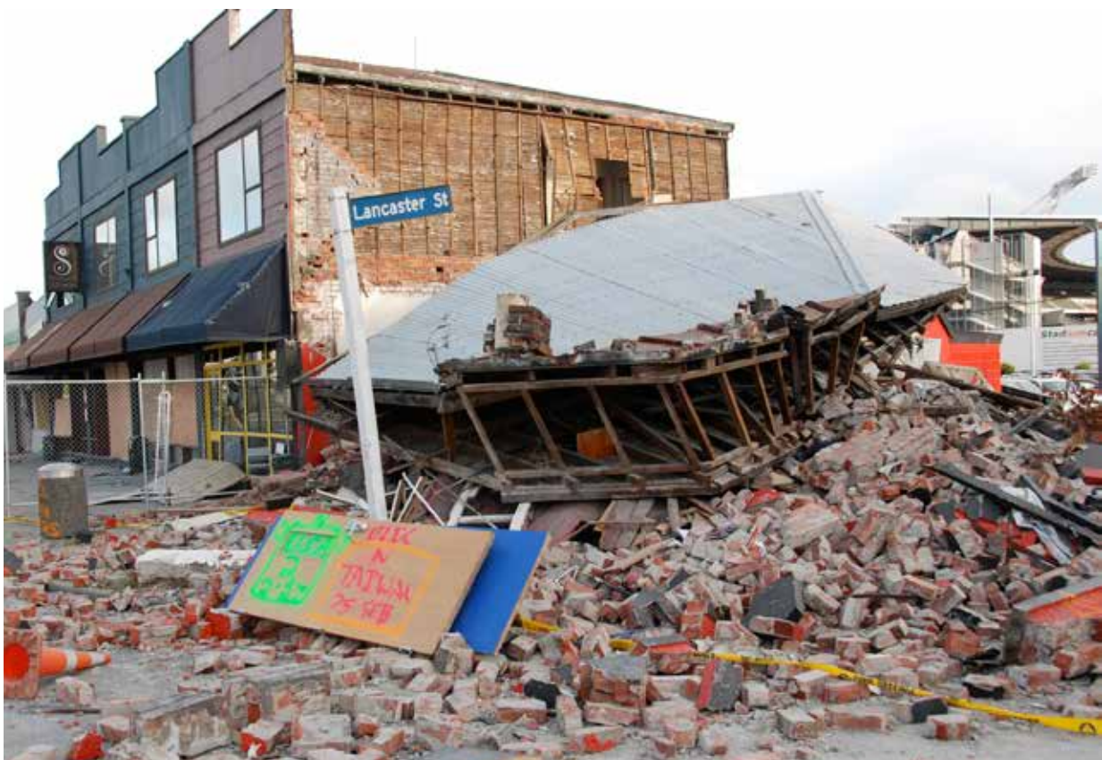
Building checked by Taiwanese urban search and rescue team February 2012.
