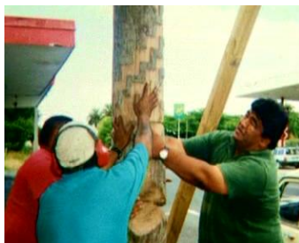
Moerewa residents erecting mainstreet veranda pou (poles)
