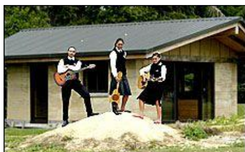
First papakāinga building made of flax fibre-reinforced rammed earth 248
