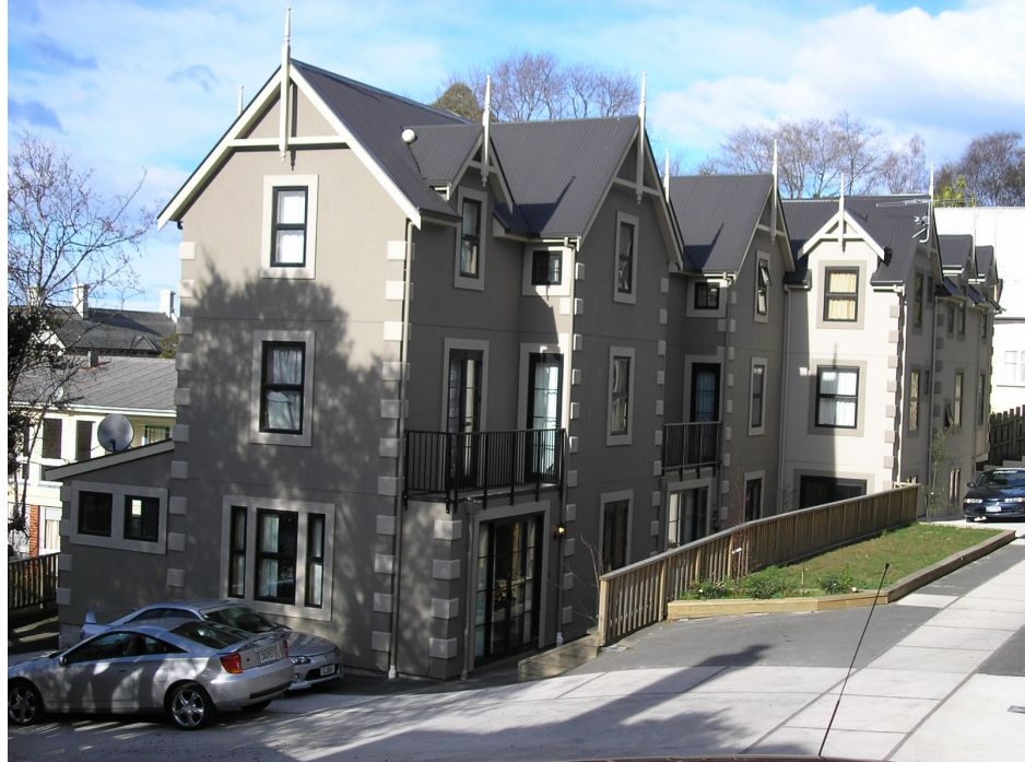
Figure 4.10: An example of intensification that has maintained heritage values in the Residential 3 Zone, North Dunedin. Source: Personal Collection, 2007.
