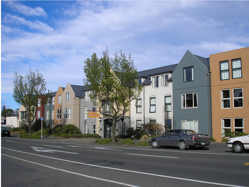
Figure 4.8: An example of ‘good’ intensification by the University of Otago, Residential 3 Zone, North Dunedin. Source: Personal collection, 2007.
